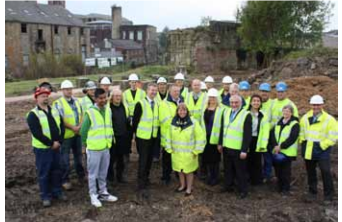
Starting work on Sandygate Square on the Weaver's Triangle, Burnley
